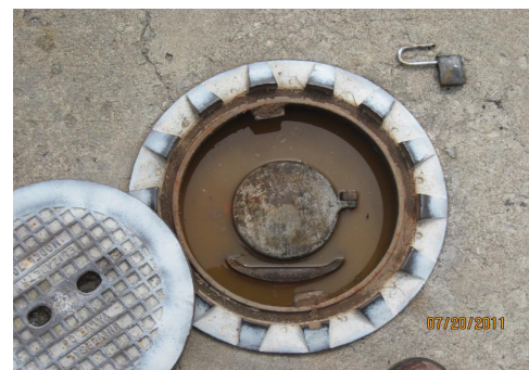
Water-filled spill bucket (Photograph by Chase Whittis)
