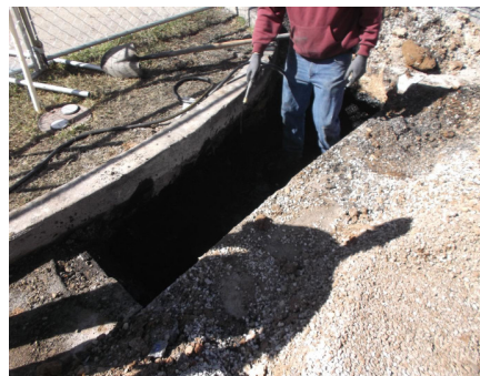
Water line excavation after repair (Photograph by Stephen Kellerman)
